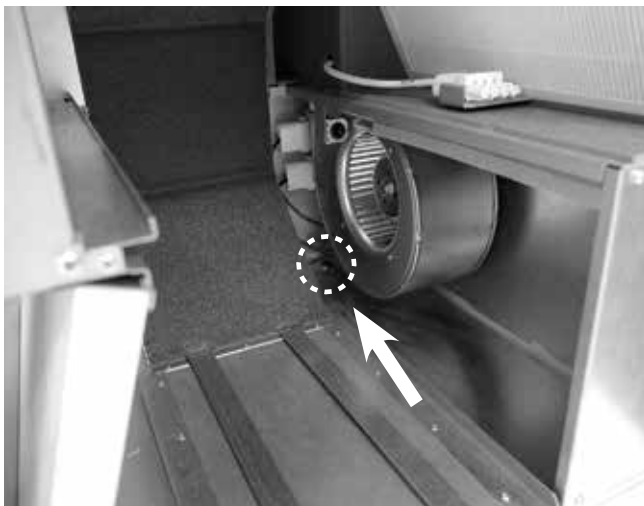
Location of the condensate discharge connection.
