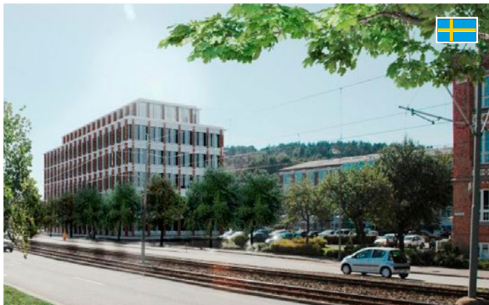
Bengt Dahlgren Head Office, Gothenburg
