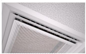
Figure 14. PD face plate Circular holes arranged in a square pattern with a graduated border
