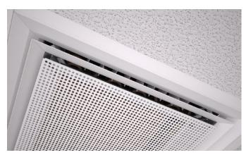
Figure 13. Standard face plate Circular holes arranged in a square pattern
