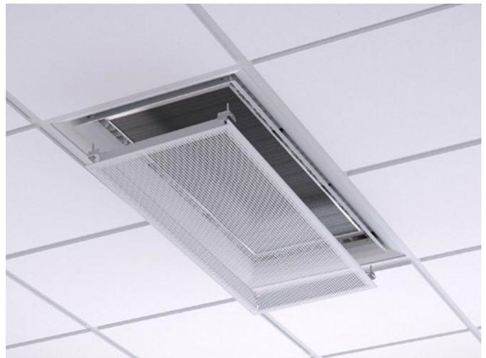
Figure 18. Removing the face plate to access the coil
