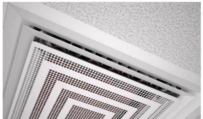
Figure 16. PX face plate Circular holes arranged in a square pattern - field perforated rectangular paths.
