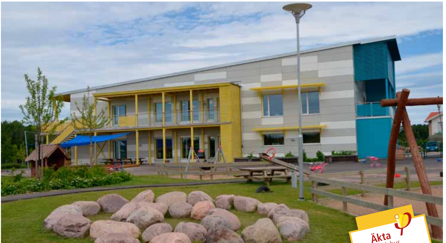
Nursery school Trädgårdsstaden in Skövde is a certified Passive House with two GOLD RX units. Photo: IG Passive House
